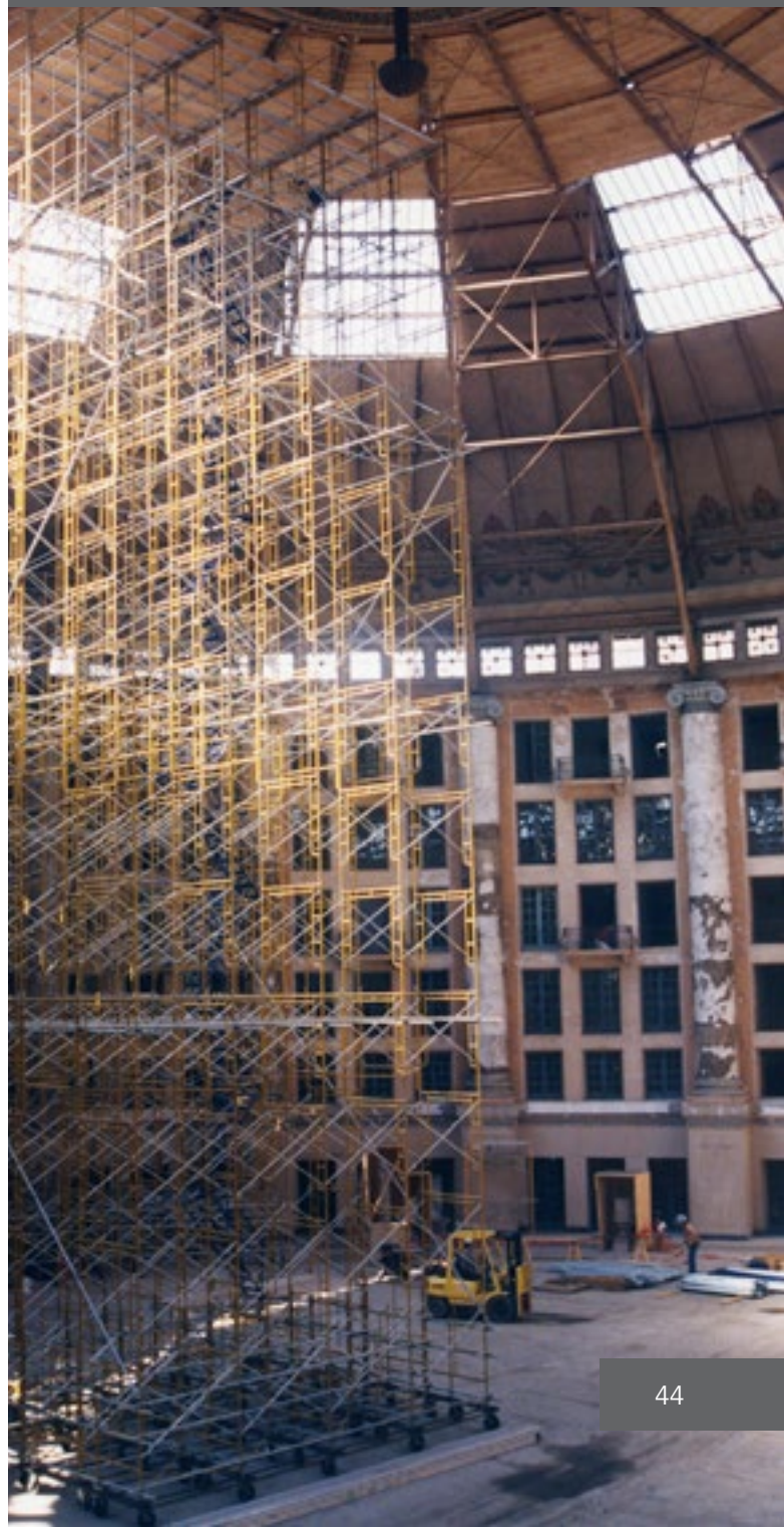
West Baden Hotel renovering
